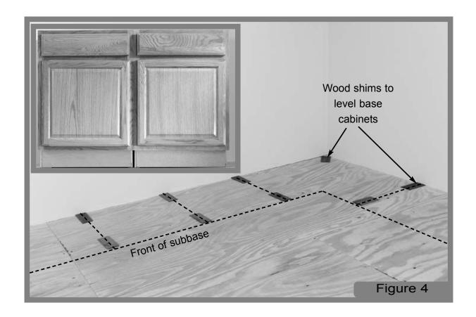
After high and low spots have been handled, ensure that cabinets hang plumb by placing a level along the vertical lines where cabinets join together and tack shims where needed. (Shims are not always required.) Shims should not stick out below or past the run of cabinets.
