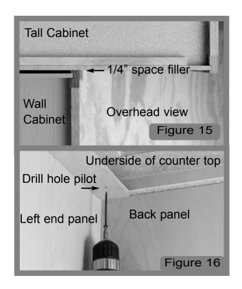
A filler trimmed to <sup>1</sup>/<sub>4</sub>" in thickness or scribe moulding is recommended to conceal the small gaps between the top of the cabinets and the soffit or ceiling.
