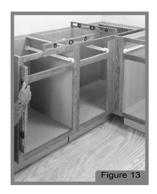
Clamp the corner cabinet and adjoining base cabinet together with the filler strip in place between them. Drill <sup>3</sup>/<sub>16</sub>" countersunk holes in the front frame of the corner cabinet. Drill pilot holes into filler and attach. Check the level of each cabinet (front to back, across and plumb, Figure 13).
